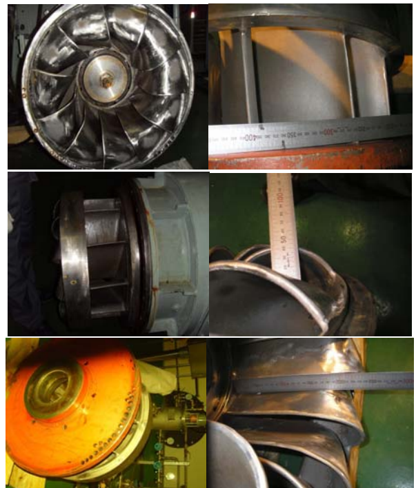
Fig. 4 Runner of the small-scale hydroturbine
