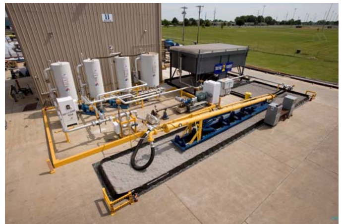
Fig.4, Aerial Picture of test facility
