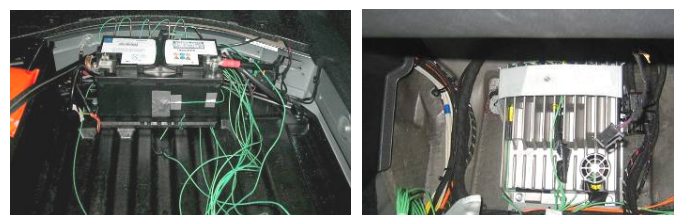
Figure 1. Back battery in the spare-wheel cavity (left) and sound amplifier in the feet compartment (right)
