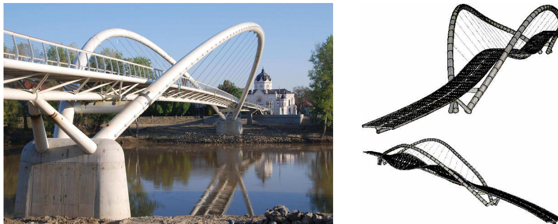
Figure 12. Picture of the investigated bridge structure and the two relevant mode shapes.
