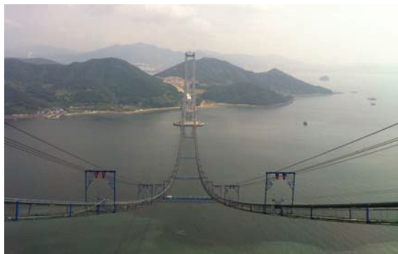
Figure 1. Catwalk structure of Kwangyang Bridge.
