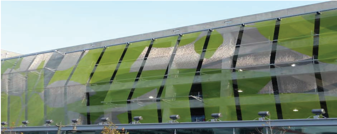
Figure 1. Exemplary Wire Mesh Cladding Structure at the Los Angeles Police Department, USA
