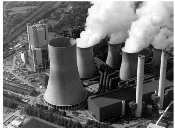
Fig. 3. Aerial view of the RWE Power Station at Niederaussem in summer 2001.
